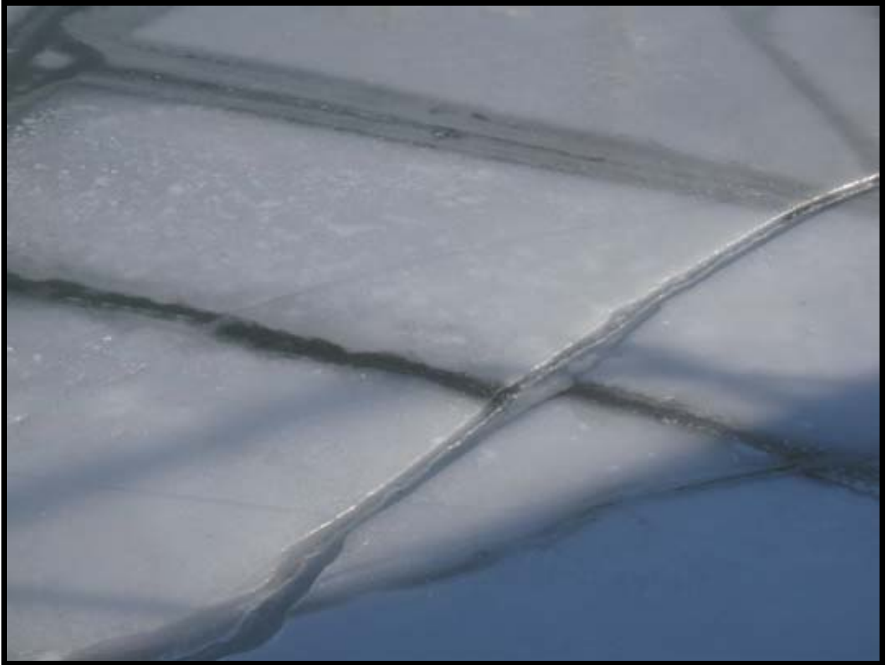
Figure 12, Cracks in the surface, digital photograph.
