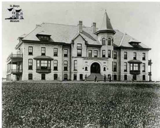
Figure 4: Perth County and Stratford House of Refuge, Stratford, Ontario, built in 1896. Spruce Lodge Home for the Aged stands on the former site of the House of Refuge. (St. Marys Museum).
